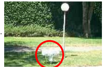
THE WATER MAIN NEAR THE BIKE PATH AND A LAMPOST
