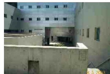
1) LOOKING OVER THE LEDGE TOWARDS THE BACK LOBBY OF SOC SCI 1100
