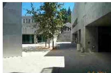
2) LOOKING TOWARDS THE WIDE STAIRS OF THE SSH BUILDING
