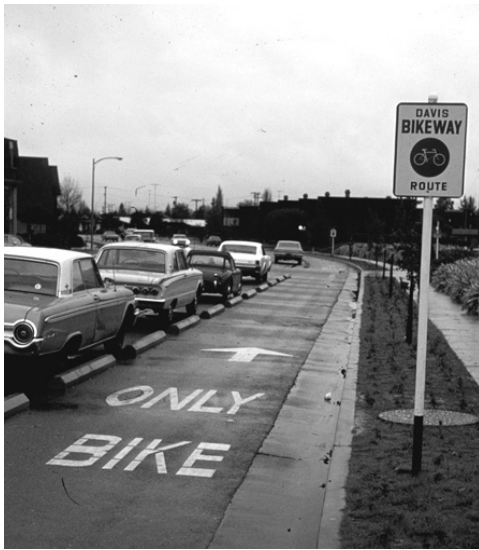
Figure 2. Amsterdam-style bike lane prototype, with one-way bike travel behind parked cars. (12)
