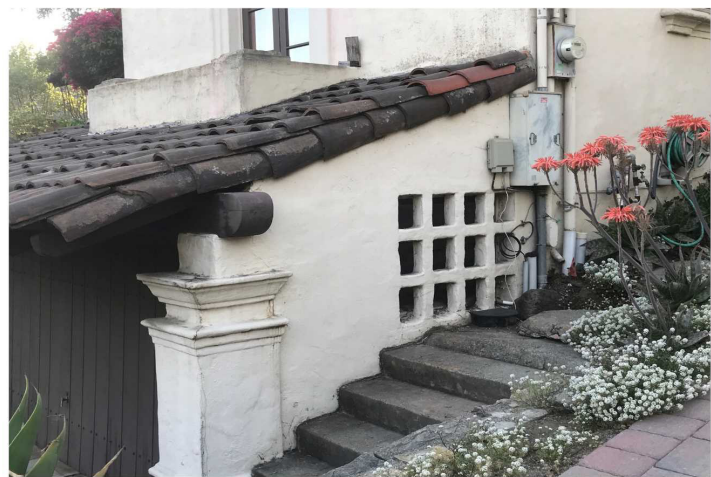
Garage window facing east
