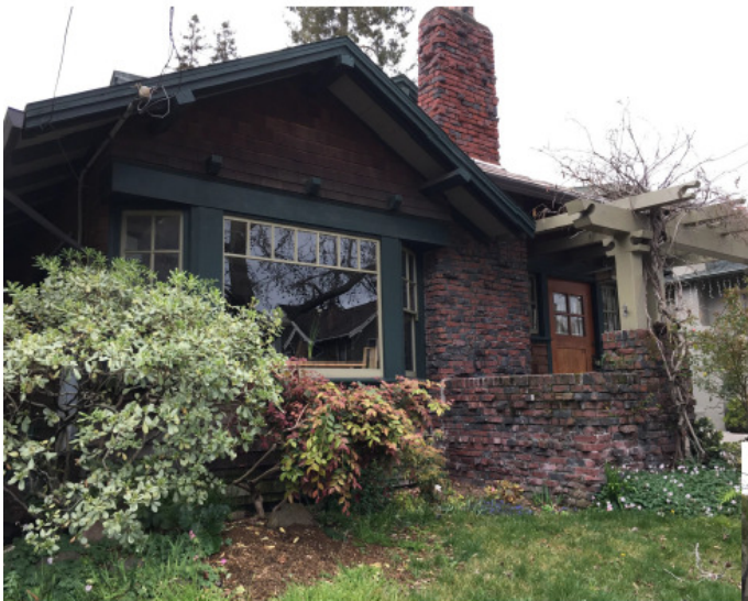
The clinker bricks in the half-wall supporting the trellis were removed from the rear of the 6475 Colby St. house. Those on the chimney are presumed to be original.
