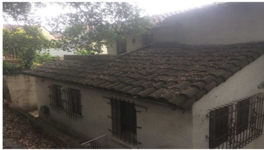
Bedroom porch occupies the visible notch on the roofline at left.
