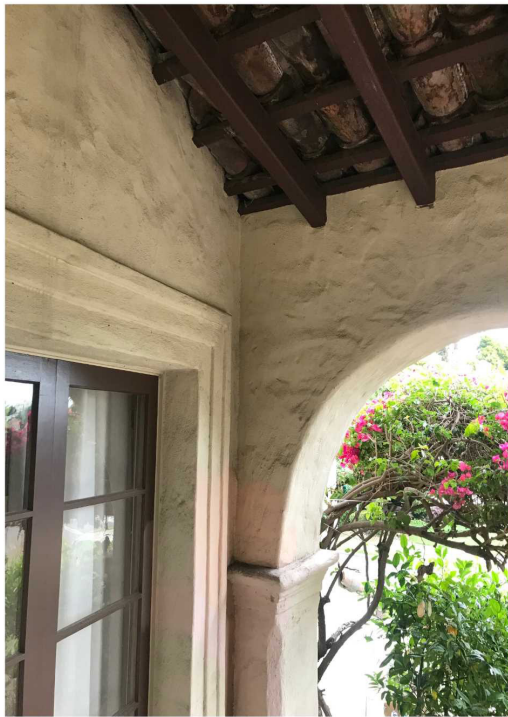
Rough textured stucco walls are trimmed out with more smoothly run cement-plaster moldings. Schirmer makes ample use of moldings to articulate features of the house and lend a sense of refinement.
