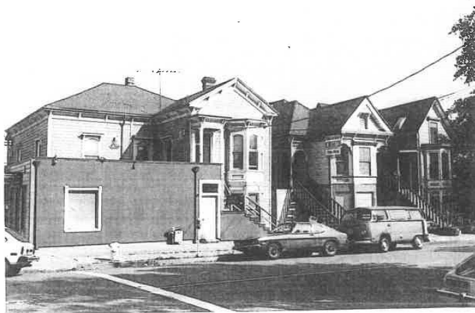
201-30A Bret Harte Boardwalk: (Jefferson St. elevation)
