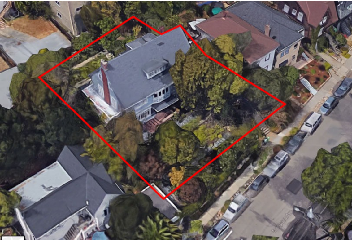
Exterior: South Front and West Side View – Google Maps, 2019
