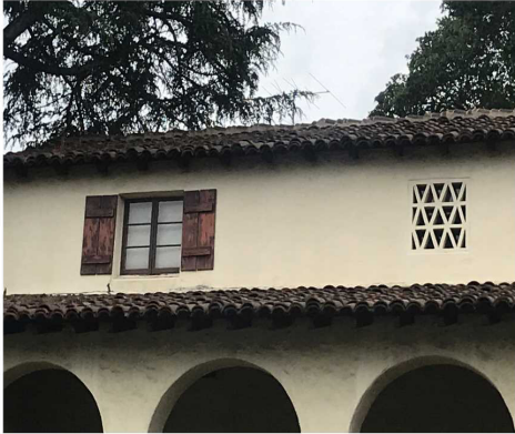
Master bedroom window, with shutters. Master bath window is hidden behind latticework which is cleverly constructed using common bricks set vertically on edge.
