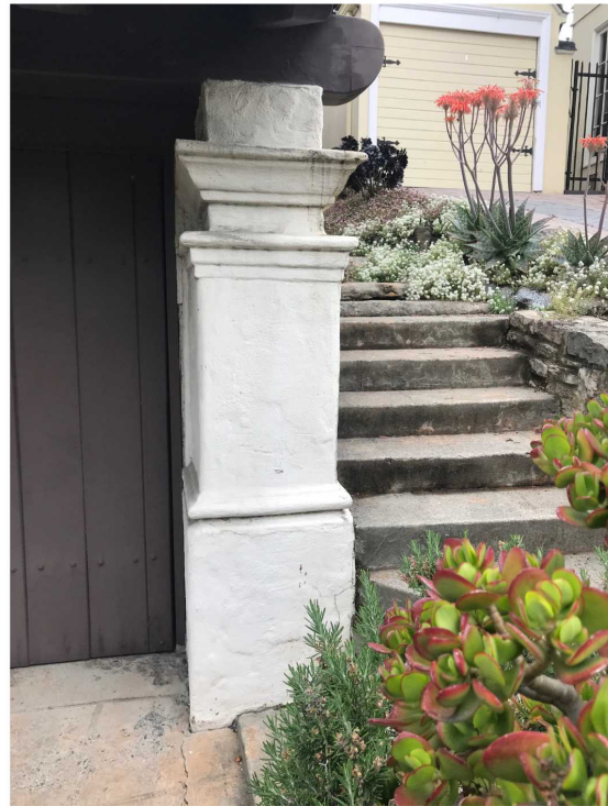
Garage entrance: Molding at top of plinth has been simplified vis a vis Schirmer's drawing.
