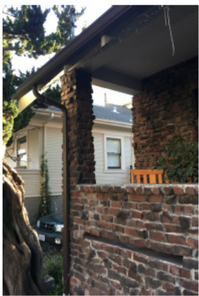
Clinker brick veneer SE corner
