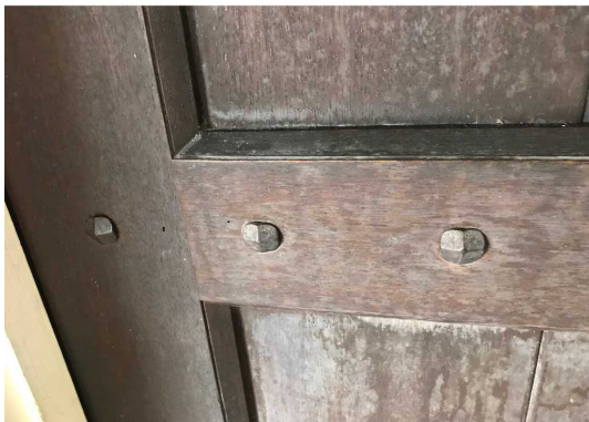
Detail of stud heads in entrance door.
