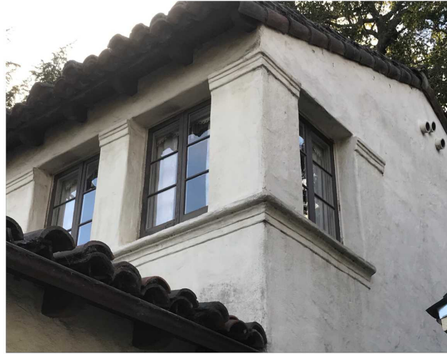
Grouping of windows in bedroom 2.
