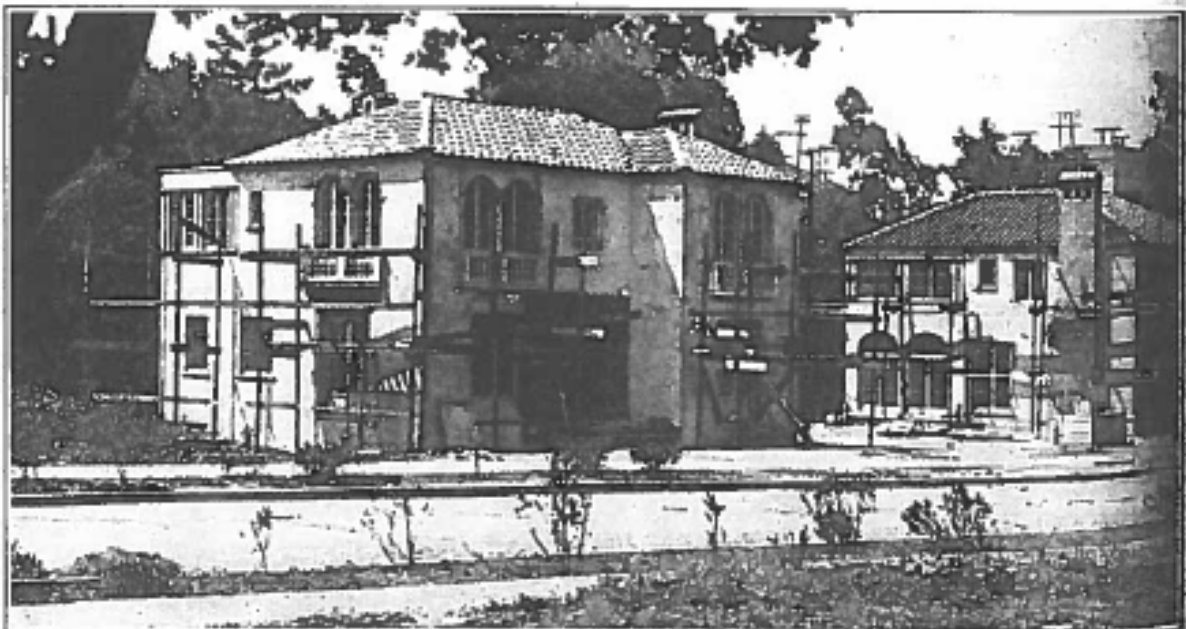
Two of the Exposition Homes in course of construction
