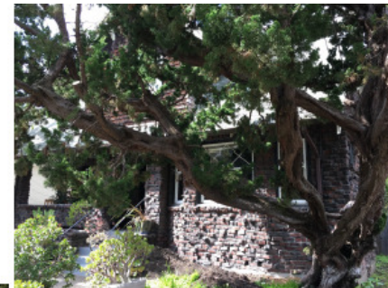
Northeast corner lot line
