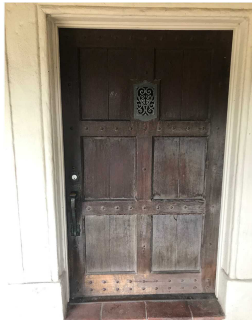
Garage entrance: Molding at top of plinth has been simplified vis a vis Schirmer's drawing.
